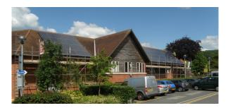
Installing the last few of the 80 panels on the roof overlooking Market St. There will be further panels on the two wings behind the main façade.
